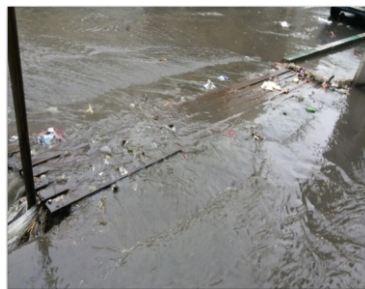
Fig. 1 : Street pollution due to clogged water channels
